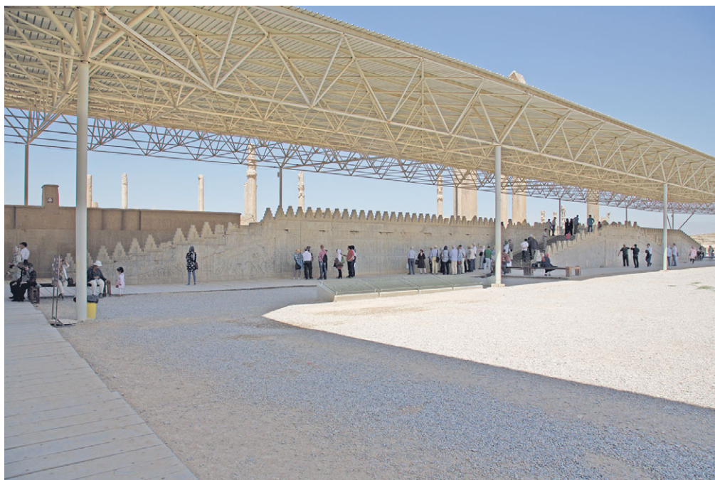
4.6. Protective roof, constructed in the 1990's, above the eastern façade of the Apadana or Audience Hall, 2009. Photo: Author
